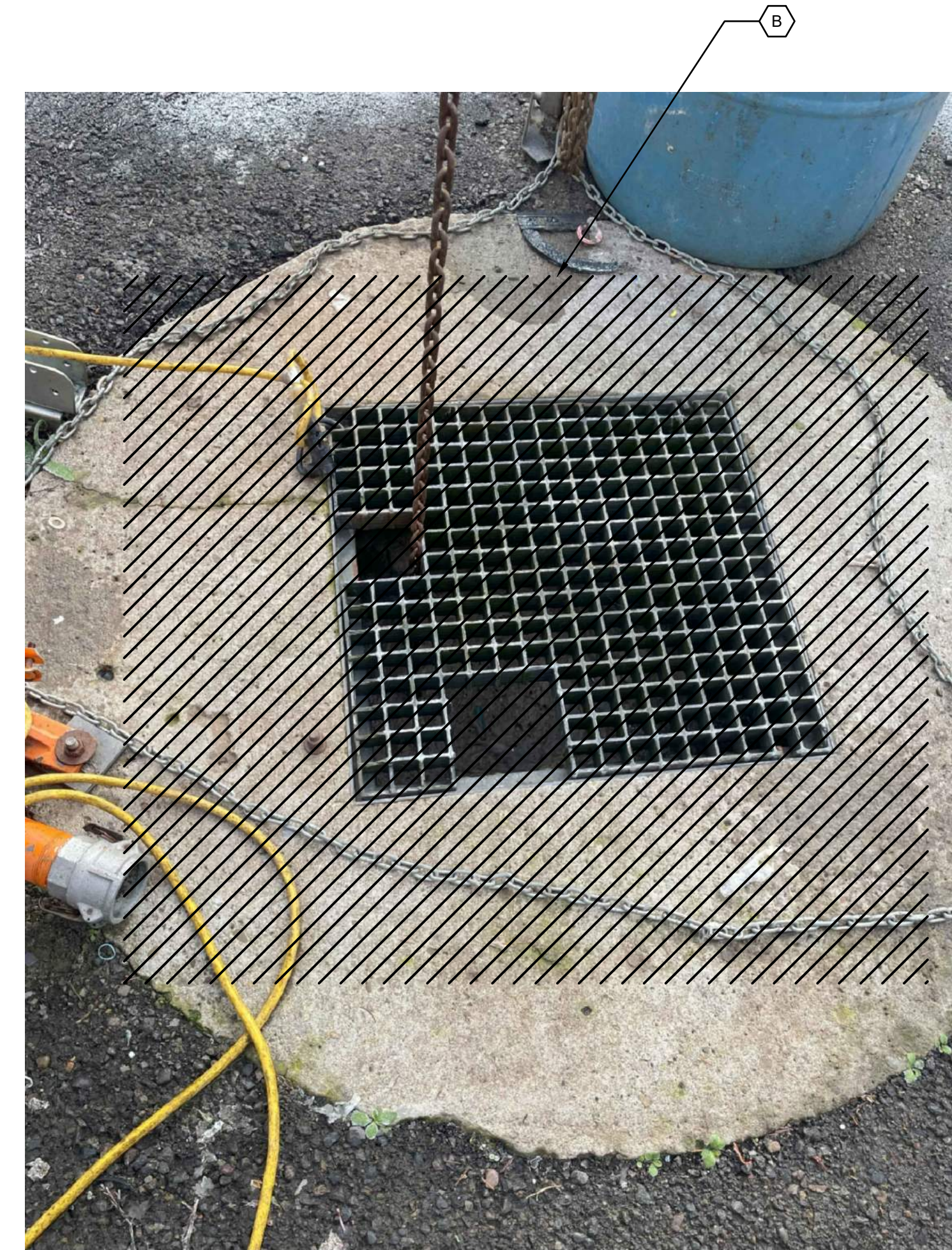
PHOTO - SCUM PIT GRATING DEMOLITION NO SCALE
