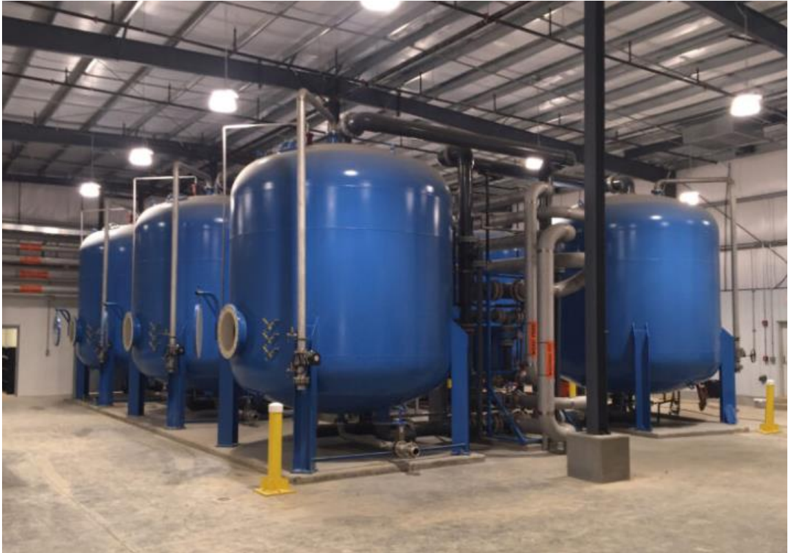
Figure 10-14: Typical GAC Treatment System
