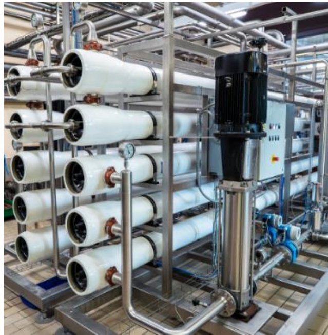
Figure 10-15: Typical RO Treatment System
