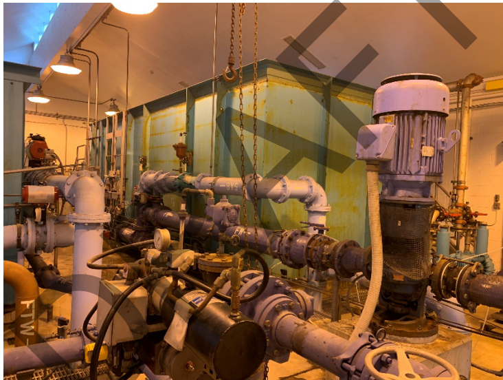
Figure 7 – Filter #3 and Single Finished Water Pump
