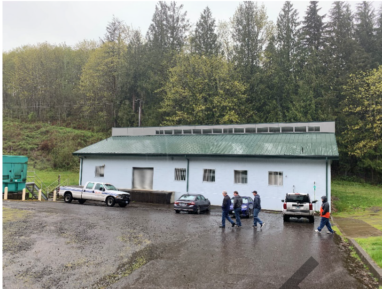
Figure 2 – Alder Creek WTP Building
