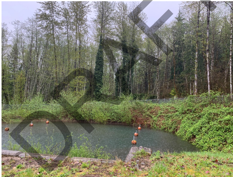
Figure 3 – Backwash Storage Pond
