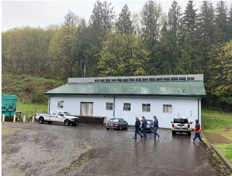
Figure 2 – Alder Creek WTP Building
