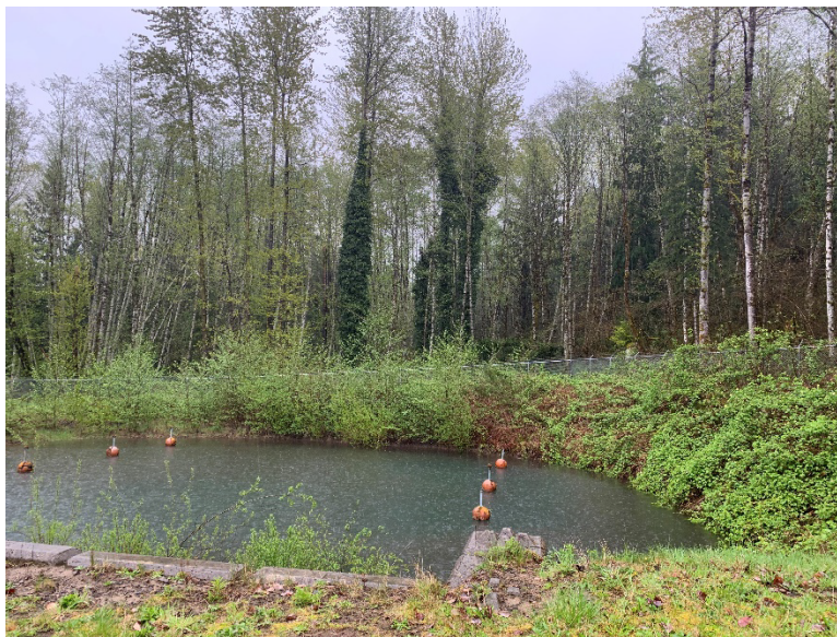
Figure 3 – Backwash Storage Pond
