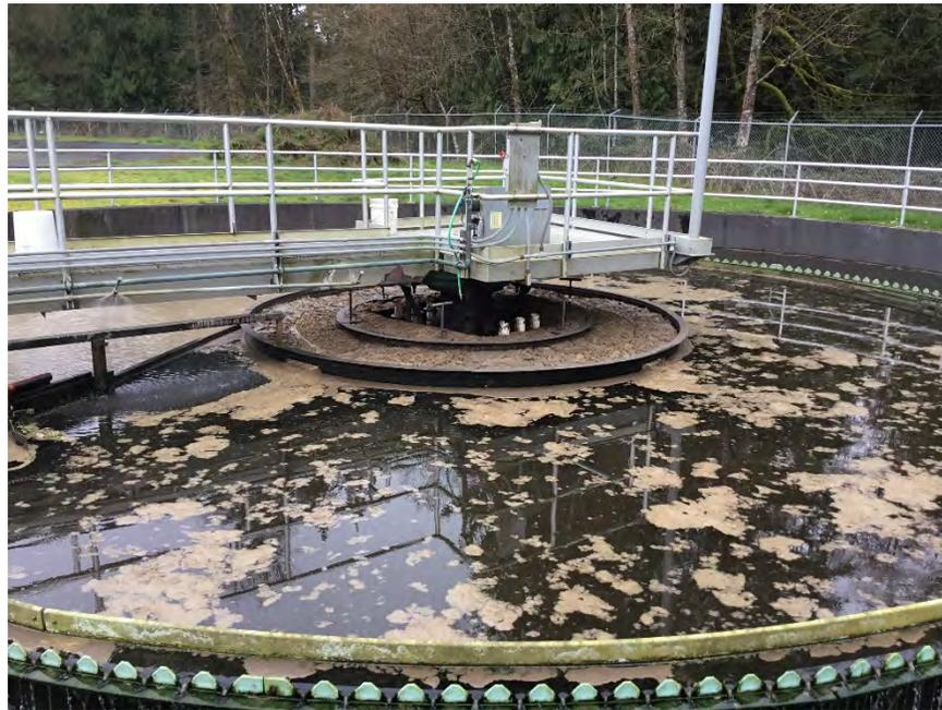
The secondary clarifiers are equipped with scum scraping mechanisms that removes scum from the surface of the clarifiers. The scum is pushed into a scum trough that drains into the scum pumping station and then gets pumped into the WAS line, which flows to the ASSB.
