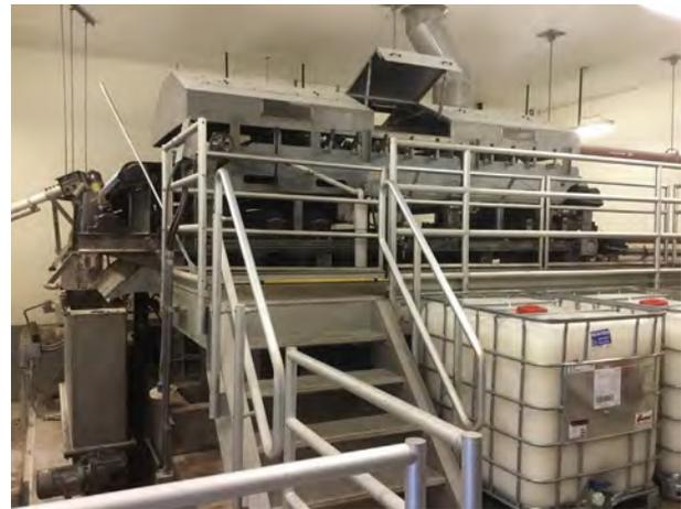
Filtrate from the belt filter press is collected and temporarily stored in the ASSB Cell #3 before being returned to the headworks facility.
