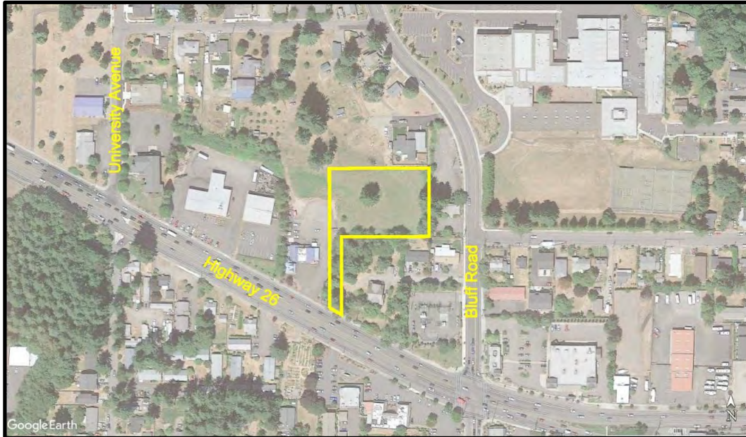
Figure 1: Aerial Photo of Site Vicinity (Image from Google Maps)
