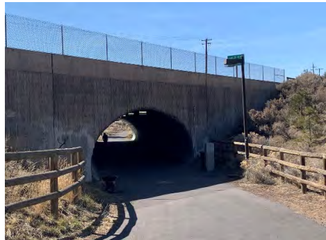
Pedestrian under-pass under Highway 20 in Bend, Oregon
