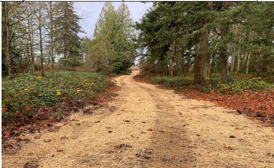
Photo 9 - Access road decommissioned January 2018, and erosion control measures complete.
