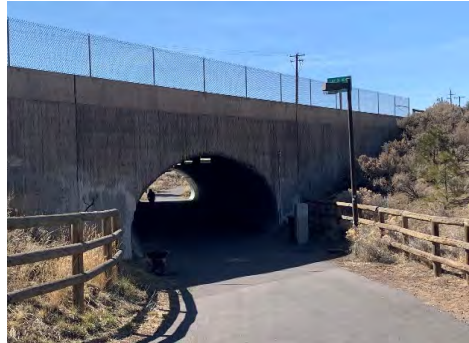
Pedestrian under-pass under Highway 20 in Bend, Oregon
