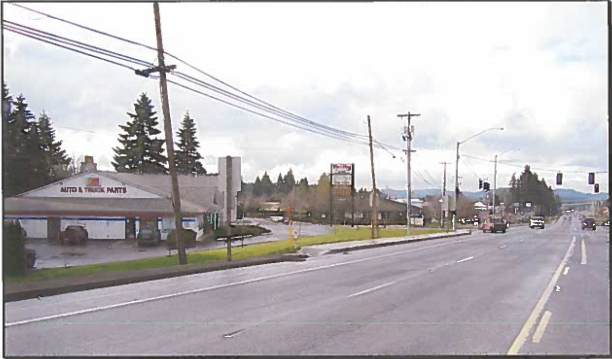
Photo 6-1A: US 26 Westbound approaching Ruben Lane - Existing Condition
