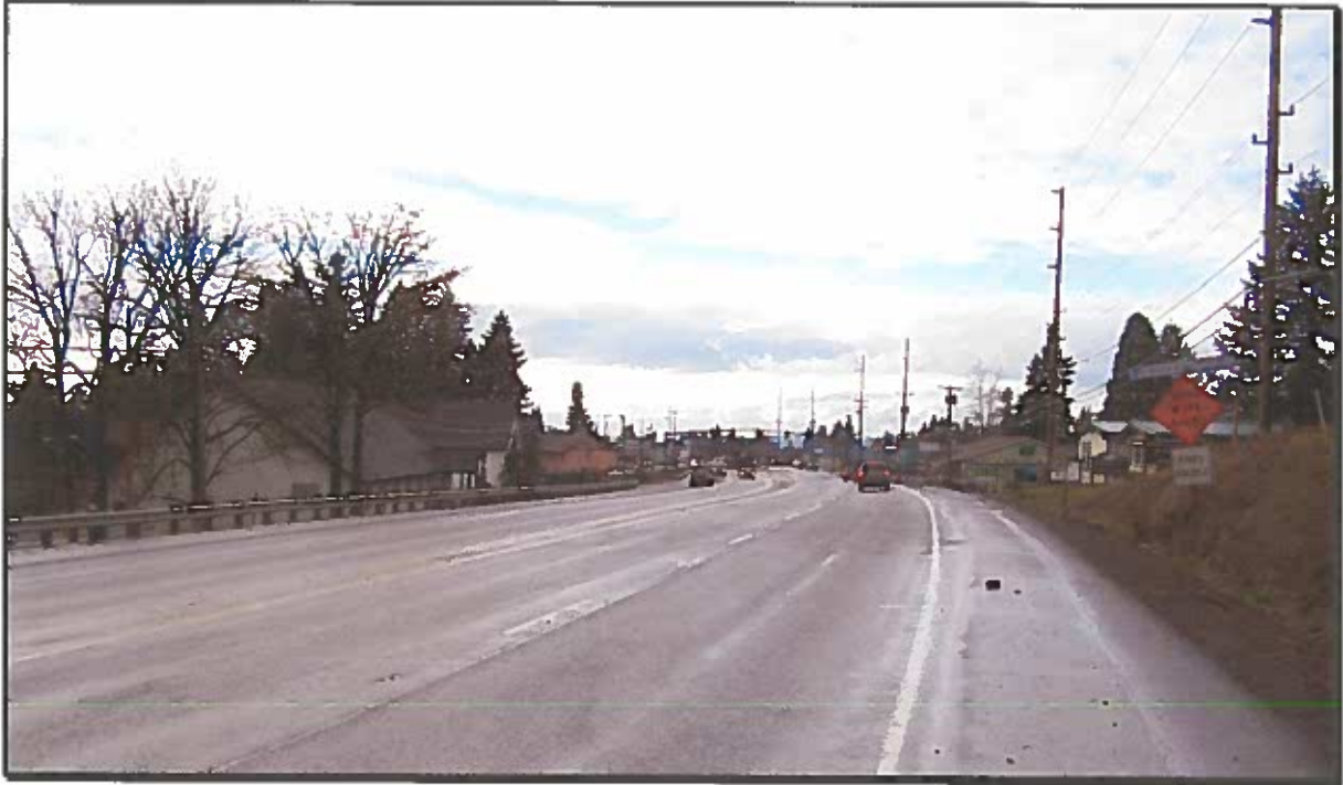
Photo 6-2A: US 26 Westbound approaching Ten Eyck Road - Existing Condition
