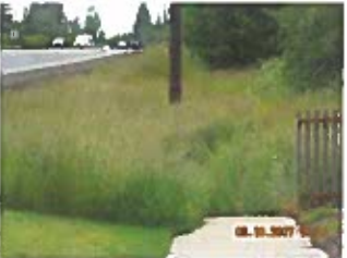
Discontinuous and Below Grade
