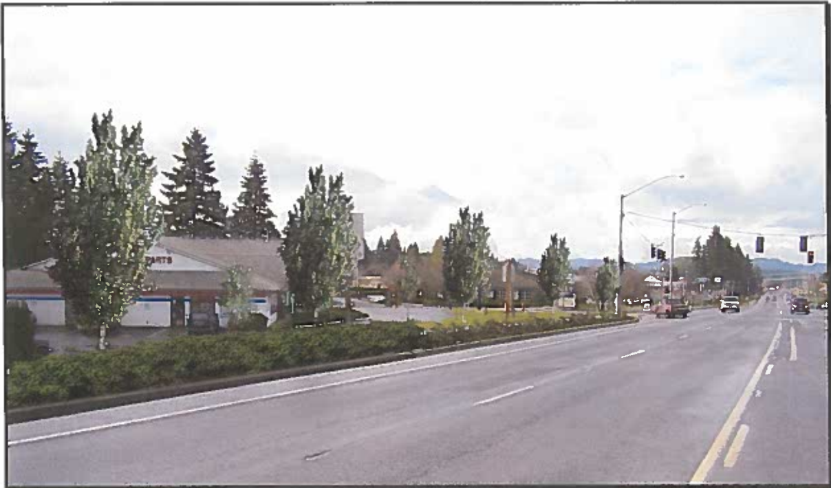
Photo 6-1B: US 26 Westbound approaching Ruben Lane - Fully Improved
