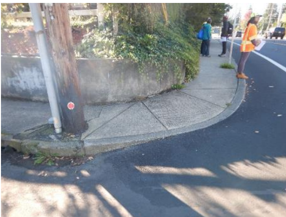
Southeast corner of Hood St and Bluff Rd, where many students cross. The intersection is lacking crosswalks, curb ramps, and some areas of the sidewalk are obstructed.
