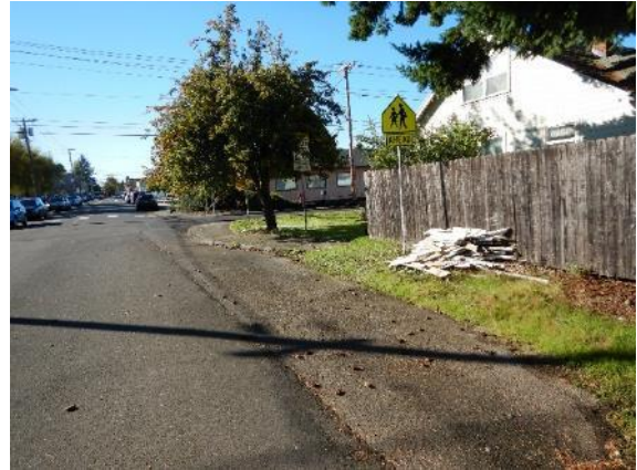
Existing southbound pedestrian crossing signage is difficult to see and placed too close to the intersection at Strauss Ave and Hood St.
