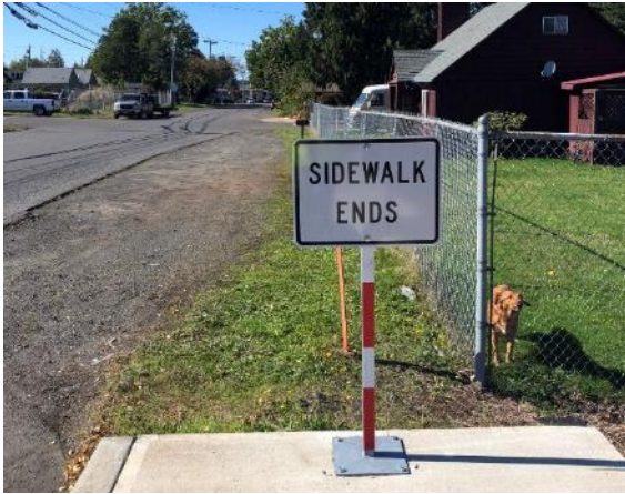
Sidewalk gap on north side of Pleasant St between Strauss Ave and Bruns Ave.
