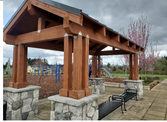
Smaller playground shelter in Bornstedt Park (12'x 20') Dog park shelter would be 14'x 20'.
