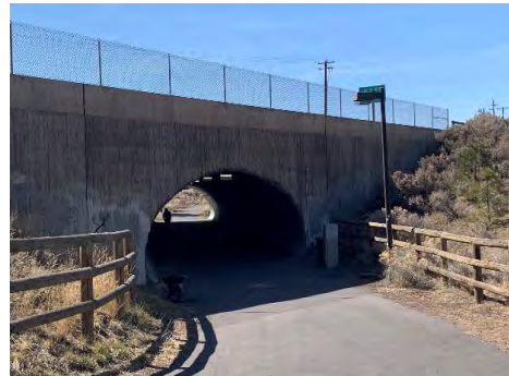
Pedestrian under-pass under Highway 20 in Bend, Oregon
