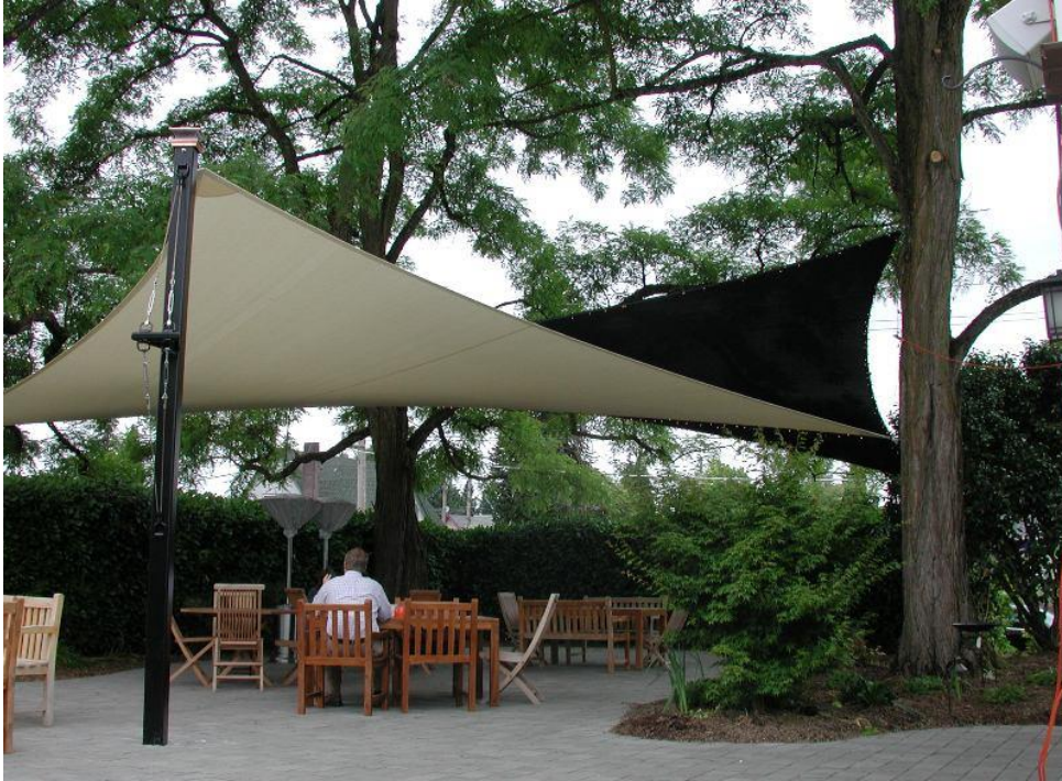
Above is an example of the “shade sail” structure canopy with middle posts ($20 to $25 per SF; For a 15' by 45' structure approx. $13,500 to $16,875).
