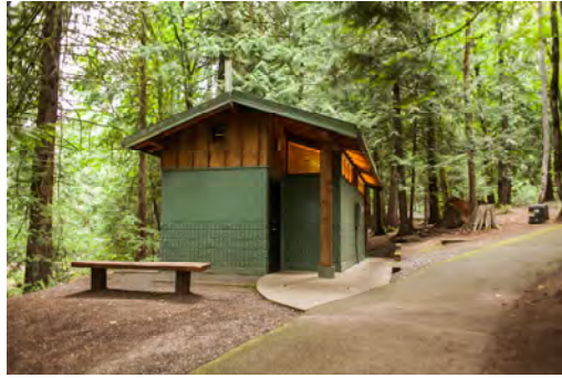
Meinig Park and Centennial Plaza host the only plumbed restrooms in the system
