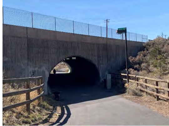
Pedestrian under-pass under Highway 20 in Bend, Oregon
