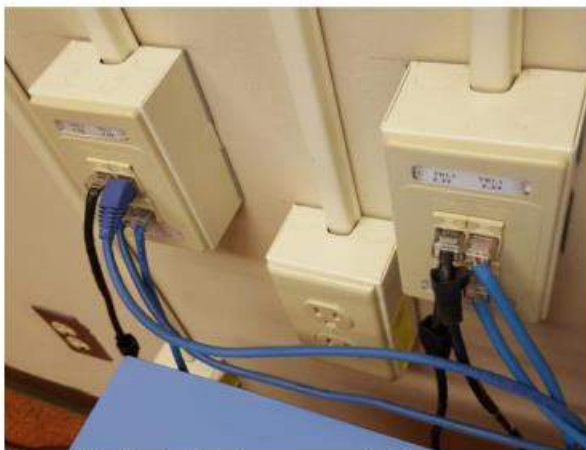
Figure E18: Typical Surface-mounted Telecom
