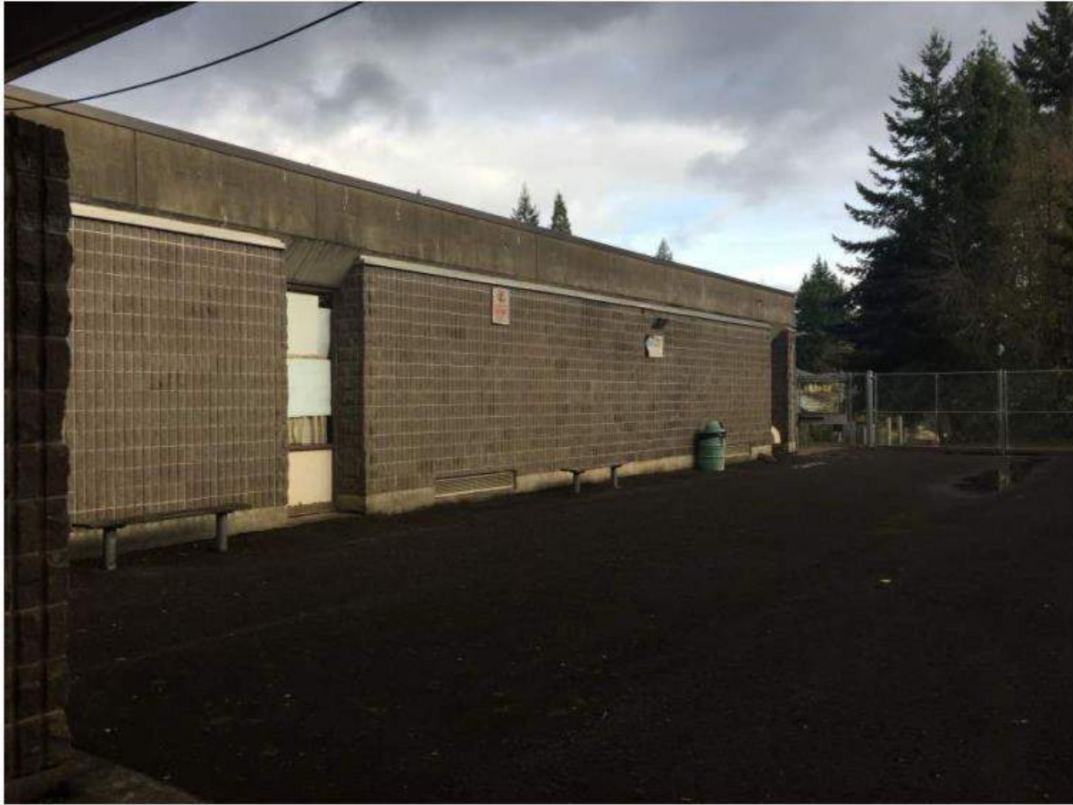
Photo 9: South Elevation – Upper School Addition.
