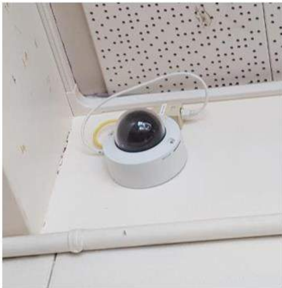
Figure E10: Typical CCTV Camera
