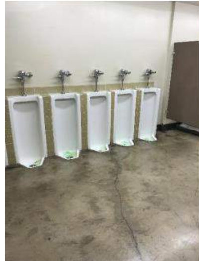
Figure P12: Floor Mounted Urinals
