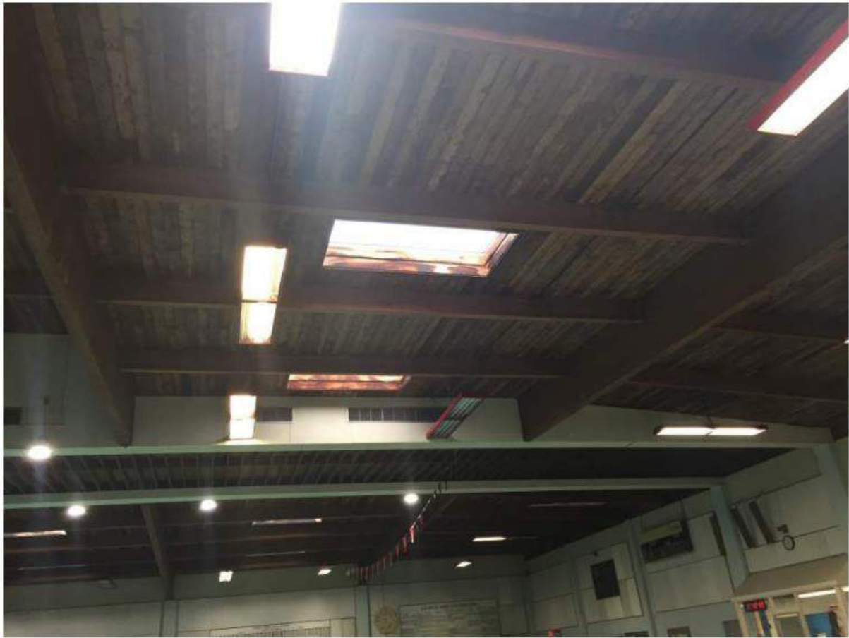
Photo 3: Underside of pool arena roof.
