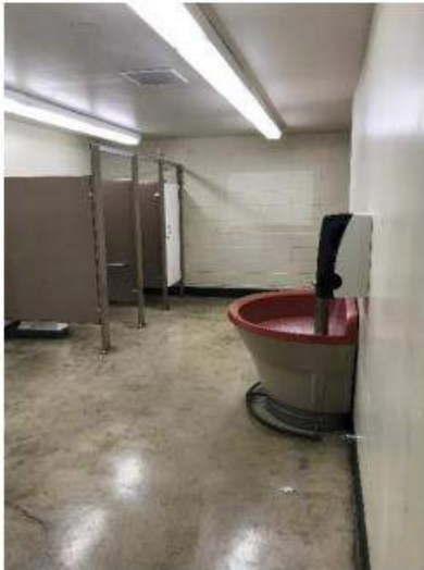
Figure P10: Existing Wash Basin
