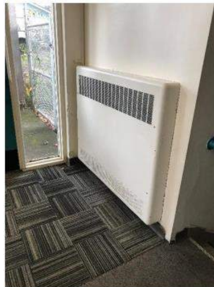
Figure M10: Steam Convectors at Vestibule
