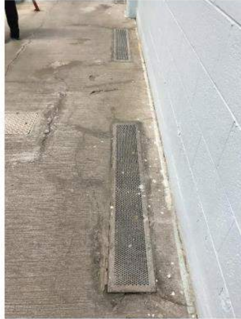
Figure M6: Pool Deck Supply Grilles
