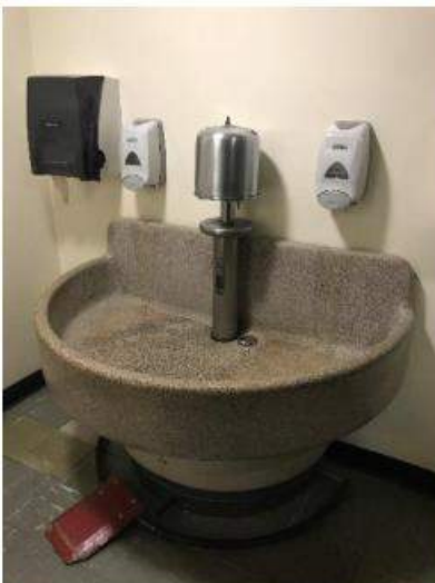
Figure P7: Existing Wash Basin
