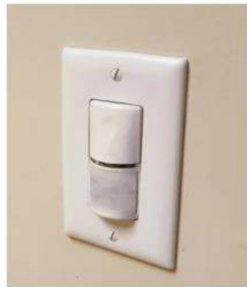
Figure E17: Sensor Switch
