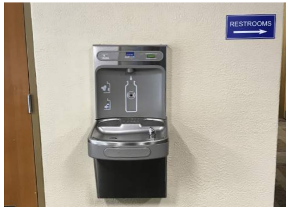
Single-height drinking fountain in lower hallway needs to be dual-height to meet ADA criteria.
