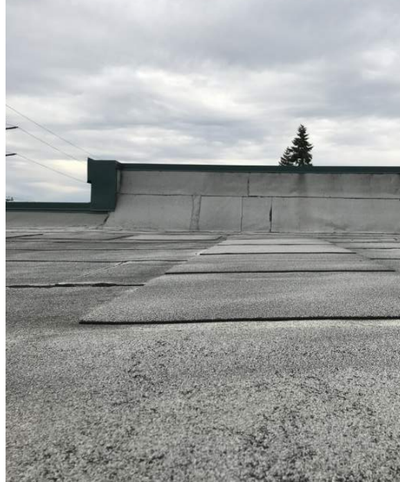
Built-up roof at Sandy Police Department.
