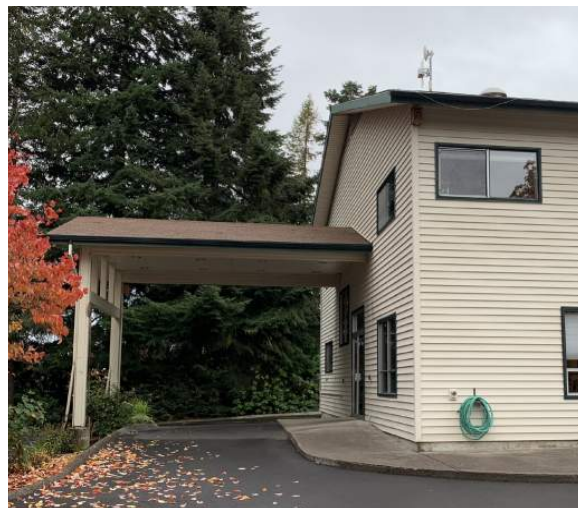
The drive-through dropoff entry is in need of structural repair or removal.
