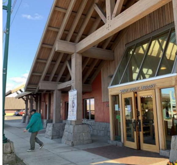
Wood elements at the Library entrance are likely to need refinishing and maintenance more often than other exterior elements.
