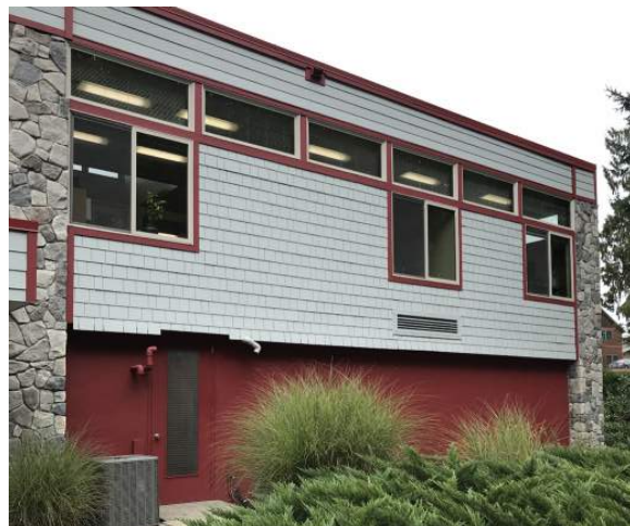
Exterior siding on south facade
