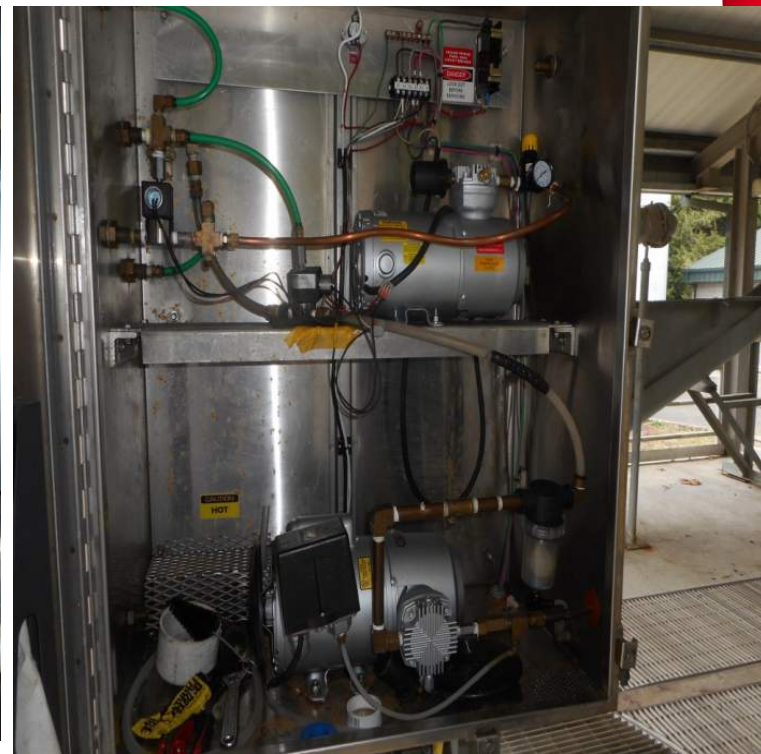
Vacuum Prime System After
