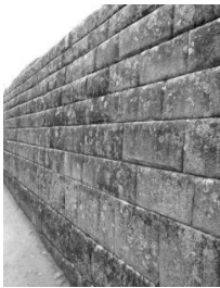
Rusticated stone work example
