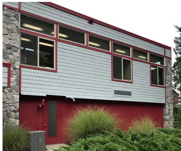
Exterior siding on south facade
