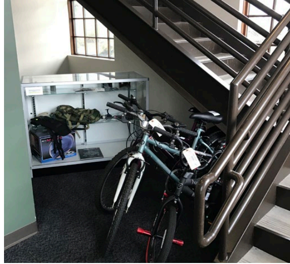
Cane detection rail should be added at under-stair locations for ADA compliance.
