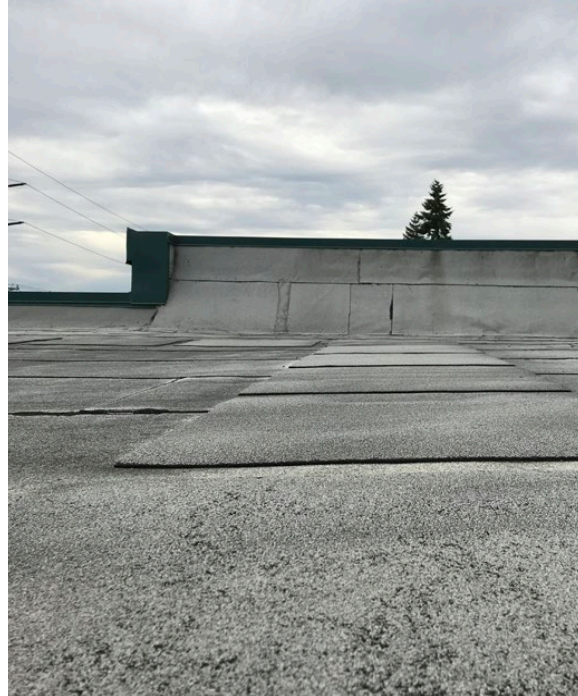
Built-up roof at Sandy Police Department.
