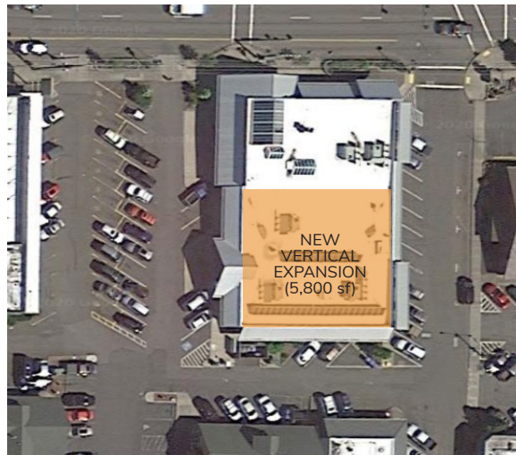
An option to build a vertical addition could allow a portion of the Library to remain operational during construction.
