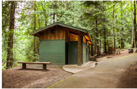
Meinig Park and Centennial Plaza host the only plumbed restrooms in the system
