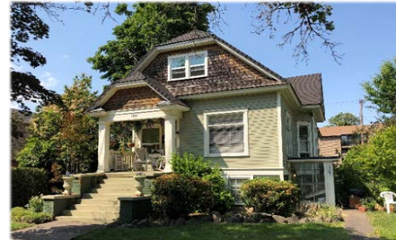
Before being outlawed, non-single-unit homes have long been built in our cities; this is a Salem triplex.
