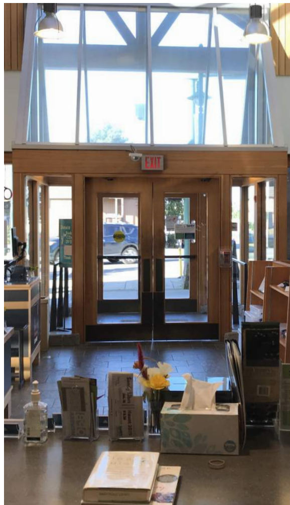
Main lobby entrance of the Sandy Public Library.
