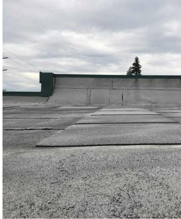
Built-up roof at Sandy Police Department.
