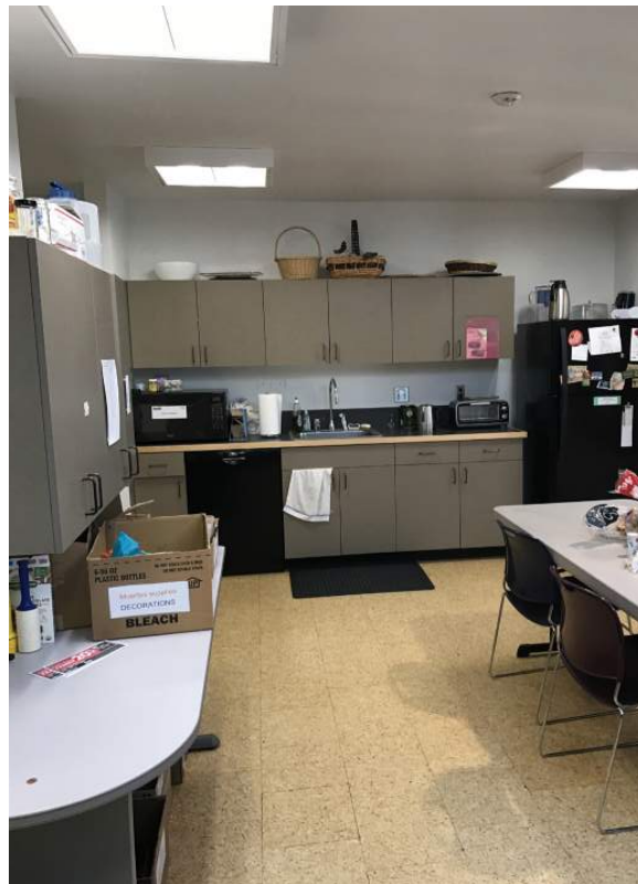
Mezzanine Break Room area is inaccessible to disabled staff.
