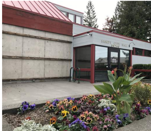
Main entry on Pioneer Blvd.
