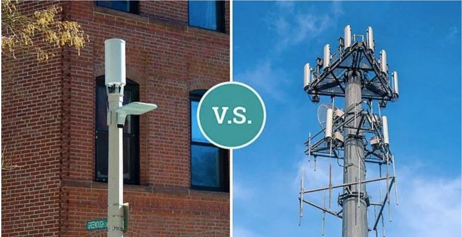
Example of small cell wireless facility versus a traditional macro tower.
