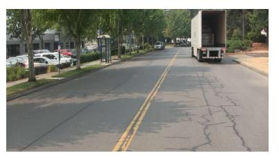
'Poor' Condition Category – Streets in 'Poor' condition are near the end of their service lives and often exhibit major forms of distress such as potholes, extensive alligator cracking, and/or pavement depressions.
