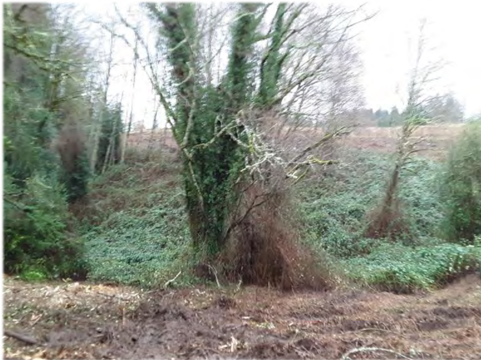
Photo Point 1. From the side slope of the ravine in the northwestern portion of the site facing southeast toward Stream 1.
