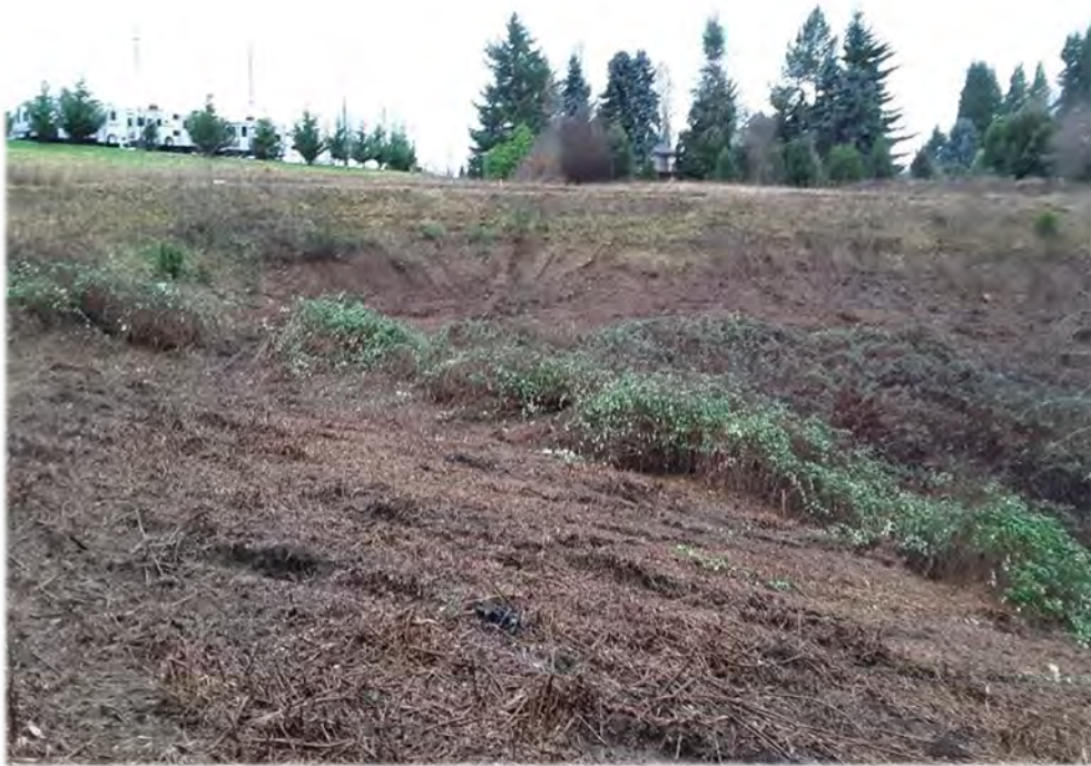
Photo Point 4. From the top of the western ravine side slope facing west toward Wetland 1.
