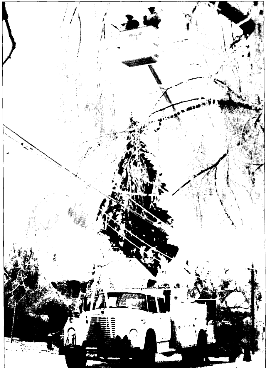
A PGE line crew works to repair damage to power lines caused by downed tree limbs during a storm.
