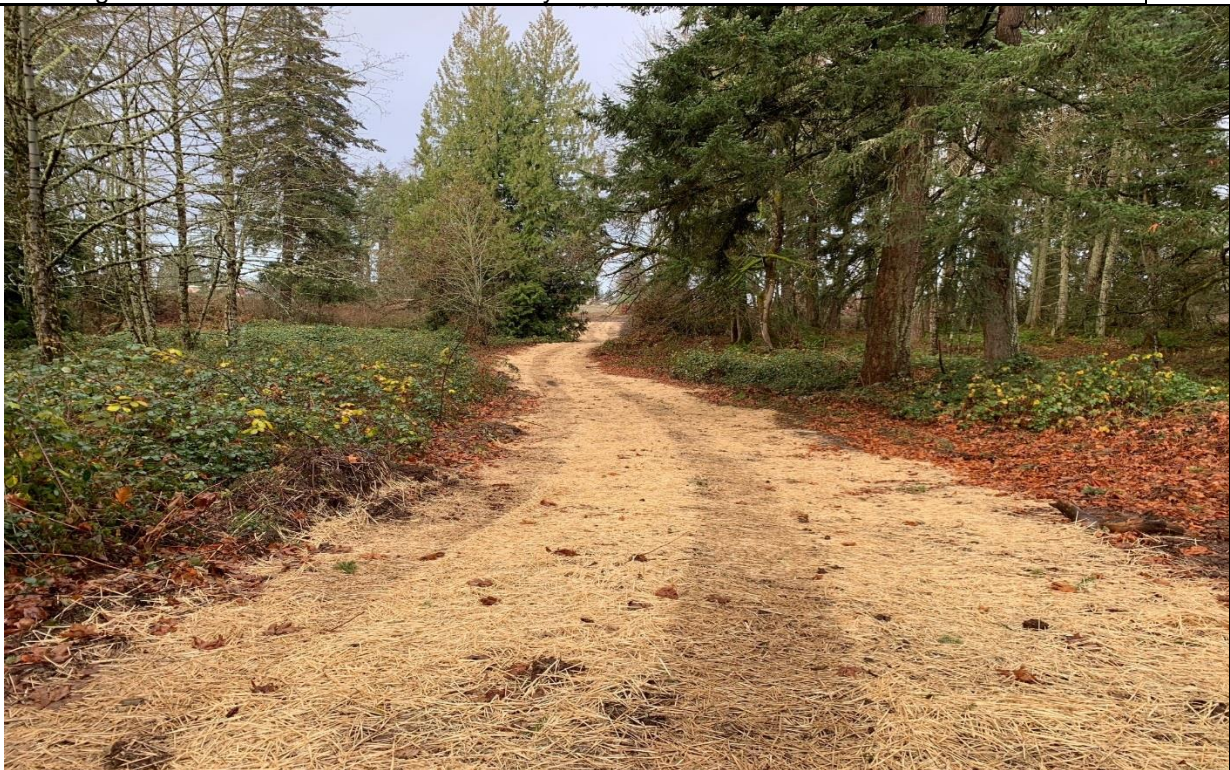
Photo 9 - Access road decommissioned January 2018, and erosion control measures complete.
