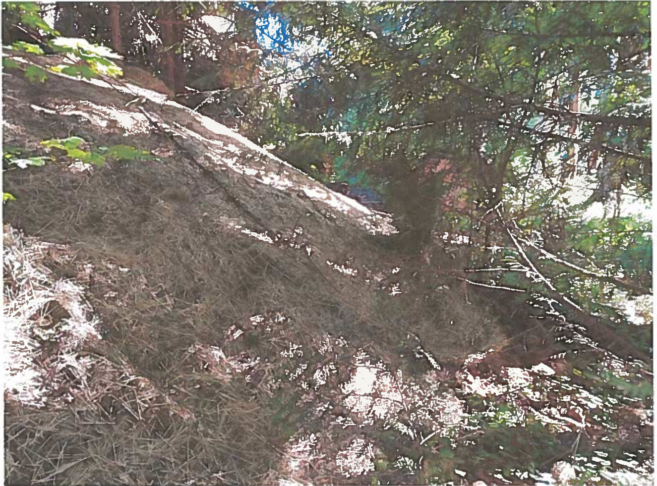
View of Fill Area, Covered with Straw to Protect from Erosion
