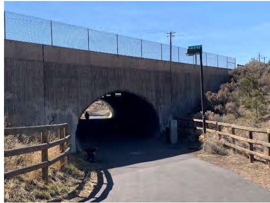
Pedestrian under-pass under Highway 20 in Bend, Oregon
